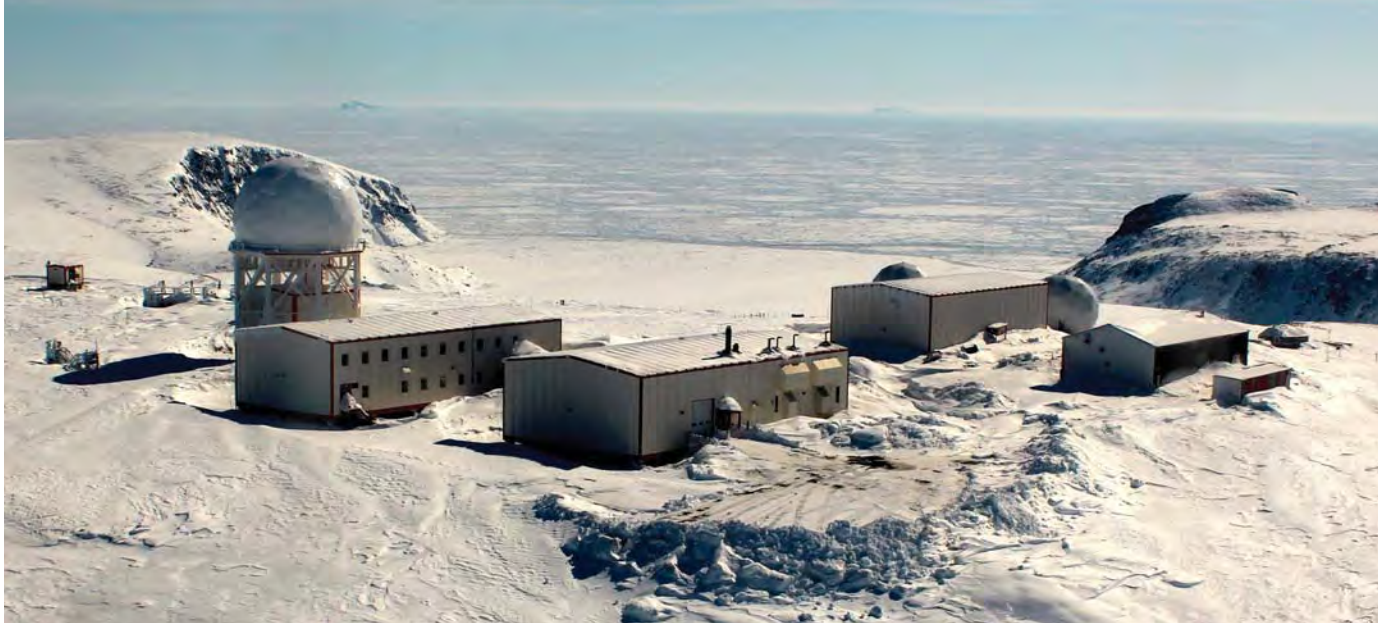
North Warning Site BAF-3 on Brevoort Island, Nunavut, is pictured in this undated photo. It was established in October 1988.
